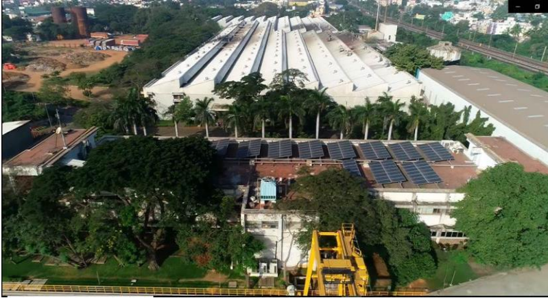
50 kWp Solar PV Rooftop Solar at Admin
